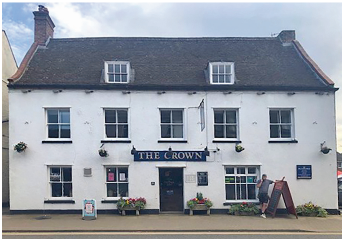
The Crown Hotel, a grade II listed building originating from the early 18th century, located on West End
