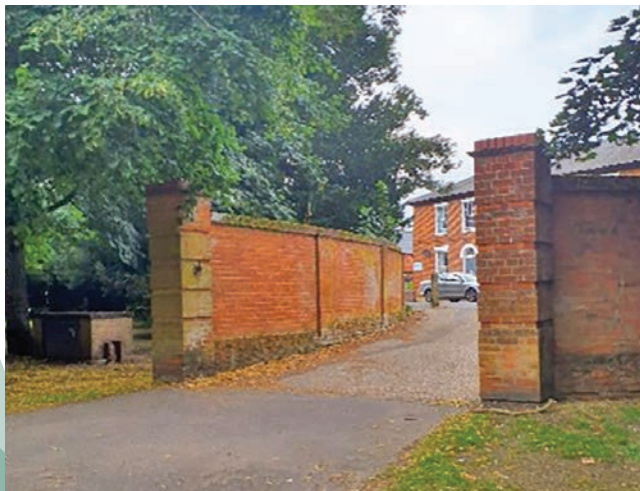
Entrance to Stukeley Park
