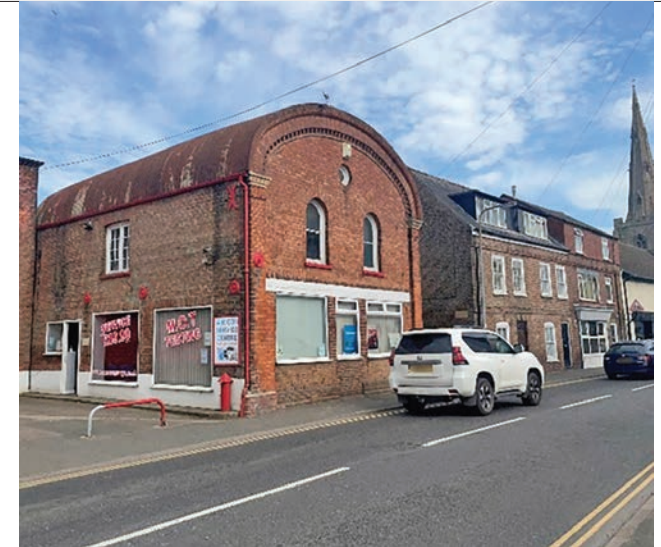
Industrial buildings, such as this example on Boston Road South, are rare within the conservation area
