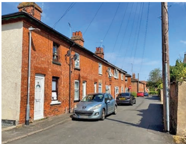
Static views within the character area
